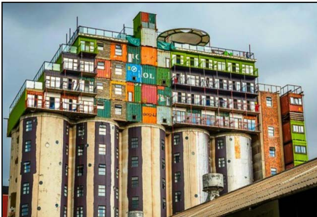
FIGUUR 8a: Citiq Property Services (Edms.) Bpk., Mill Junction , Johannesburg, Newtown, ou meule en skeepshouers, 2014.
